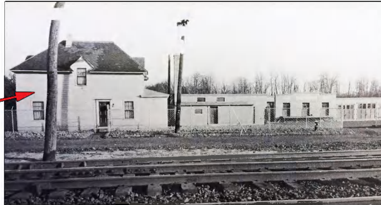
Public Works Service Building/ Caretaker's Cottage Erected 1931 at a cost of $23,565 1931 Longmeadow Annual Town Report
