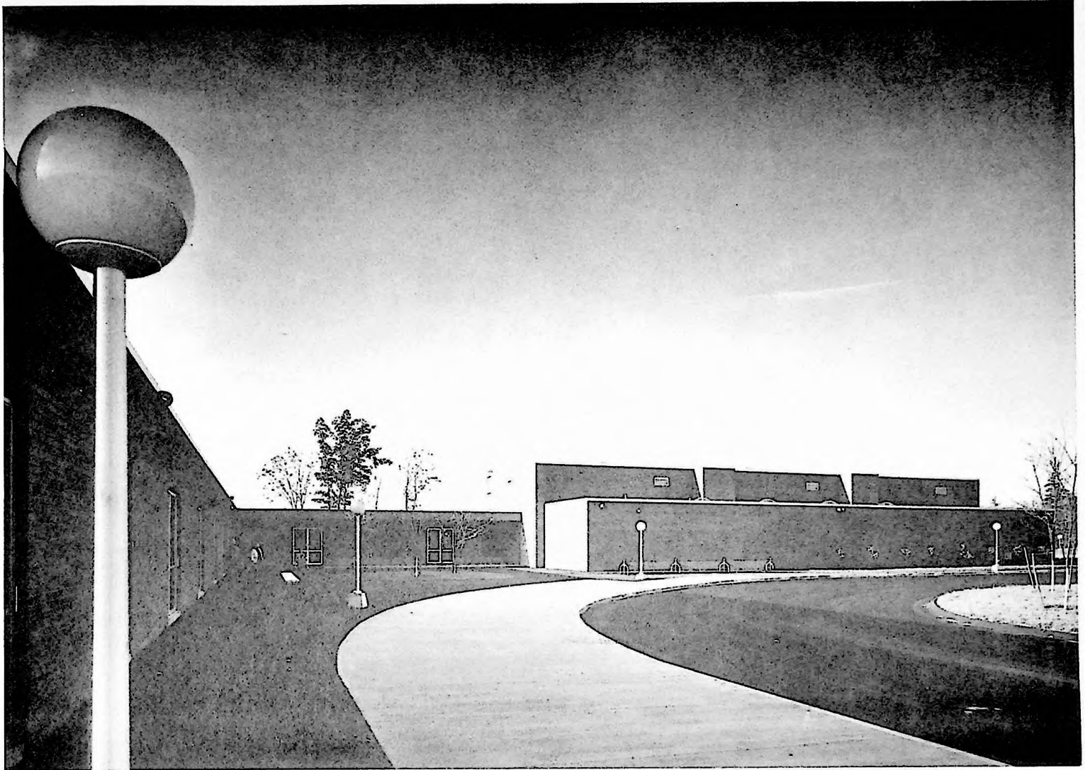
The Glenbrook Middle School, Longmeadow's newest, opened in 1968 and won an award for its architectural design.
