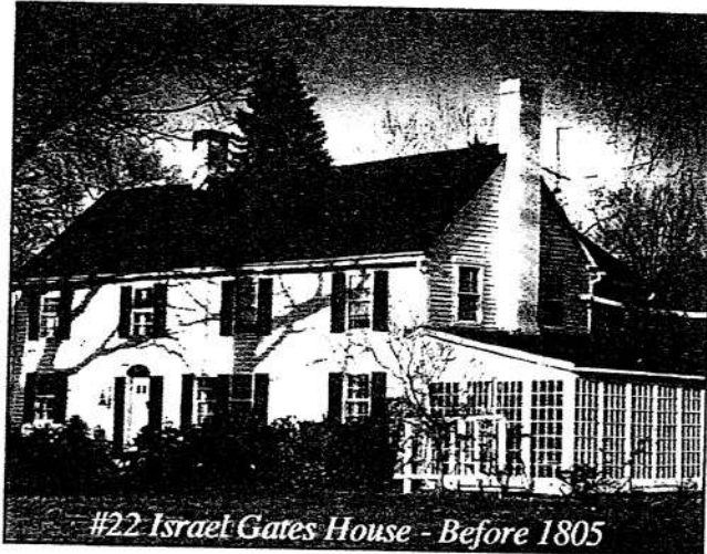
#22 The Israel Gates House - Before 1805 663 Longmeadow Street
